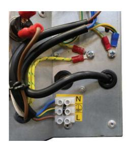
While connecting the machine to the mains power, it is raccomended to never disconnect existing ground cable. The fact of disconnecting or modifing existing cables voids the warranty and can cause troubles or accidents related to the temperature control.
